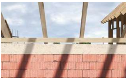
Wooden beams adjustment
